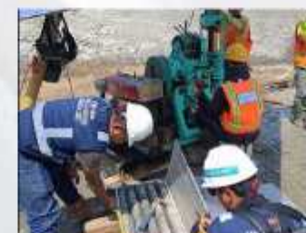
Grouting Test STA 1+590
